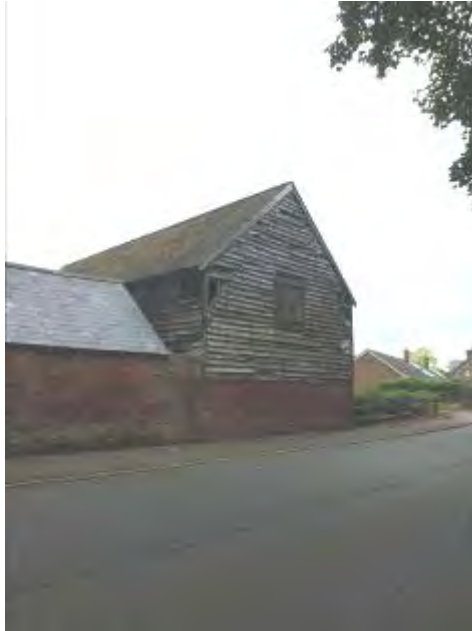
PARTS OF STONEBRIDGE FARM BUILDINGS, STATION ROAD, BEFORE THEY CHANGED
